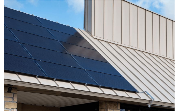
PV panels clip onto standing metal roof seam.
